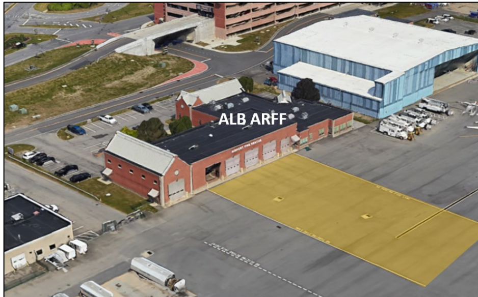
Figure 4-14 – Existing ARFF Station
